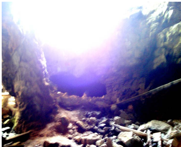
Photo 7. Queen Victoria Adit Workings
